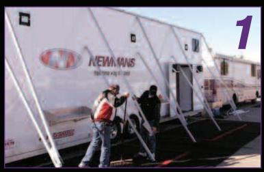
Lay-out framework and use quick connect ends to affix to trailer and supplied pins to connect A-frames.
